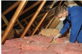
Loft insulation being laid
