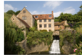
Micro-hydro power, Gants Mill, Somerset, UK
