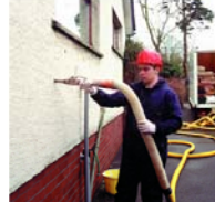
External cavity wall insulation
