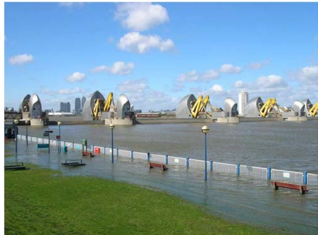
The 100th closure of the Thames Barrier. Although there is localised flooding downstream, the city behind is protected. (Photo: UK Environment Agency)
