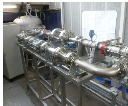
General view of the hydraulic test loop
