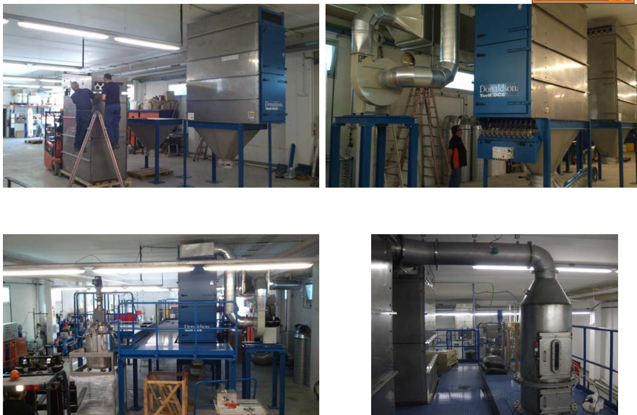
Figure 5. Installation of filters, off-gas piping, platform, burner chamber and aerosol piping
