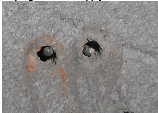
Left: Nails 3-4 in LWC concrete; right: Nails 7-8 in Thermalite
