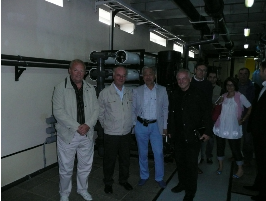
Visit water treatment plant – Astana – Kazakhstan – Mai 2010
