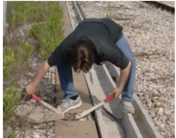
Figure 59 Unauthorized opening of the duct
