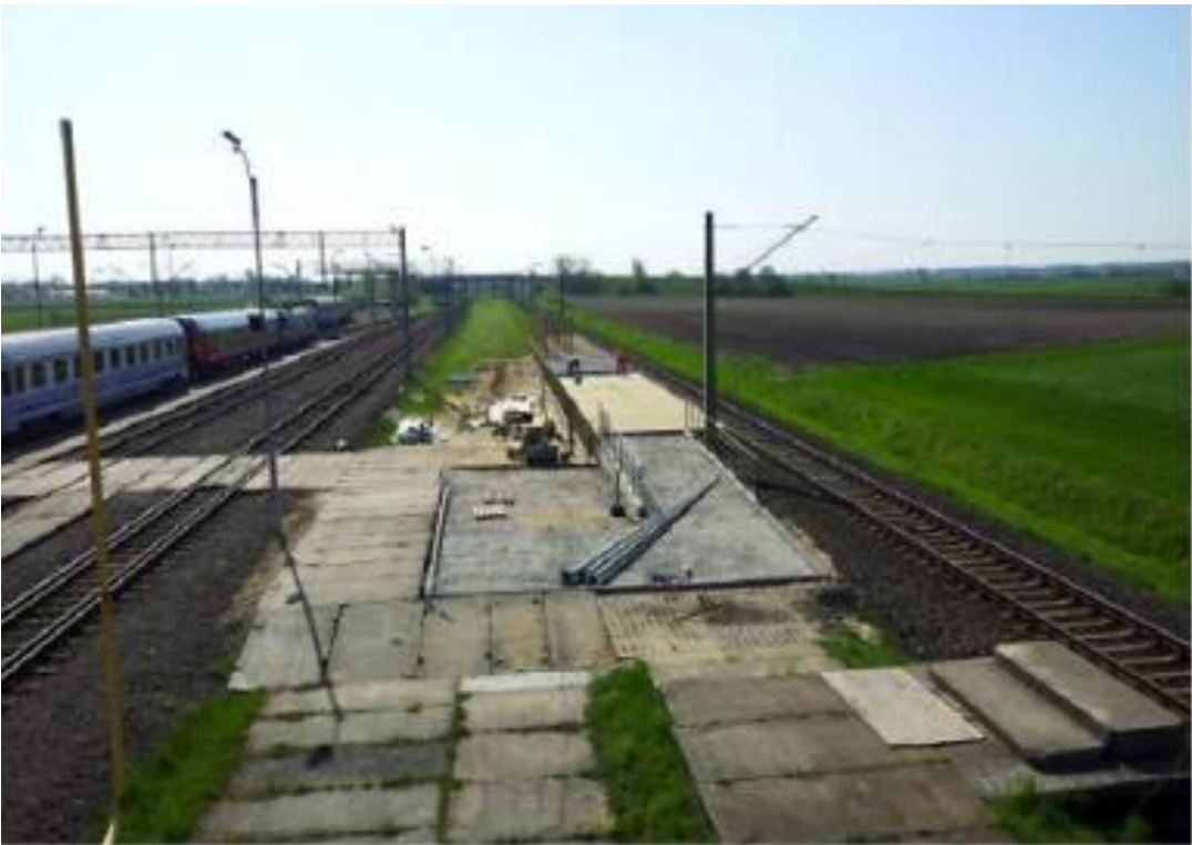
Figure 26 The Platform Construction
