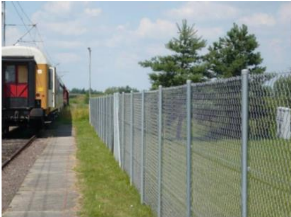
Figure 32 The installed Fence
