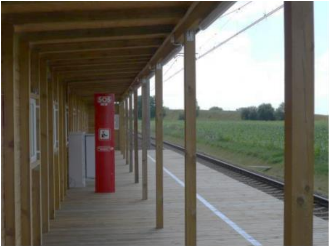
Figure 27 The platform at the end of the construction works
