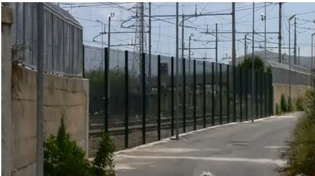
Figure 55 The active fences installed
