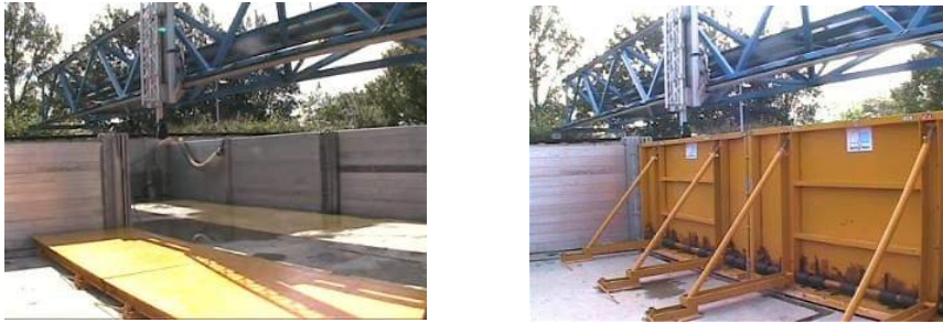
Figure 3: Spring Dam in the passive (left) and active (right) states
