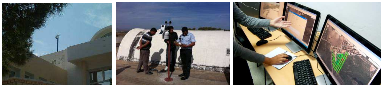
Figure 25: Camera, weather station and control centre PC installed in the Temple of Water
