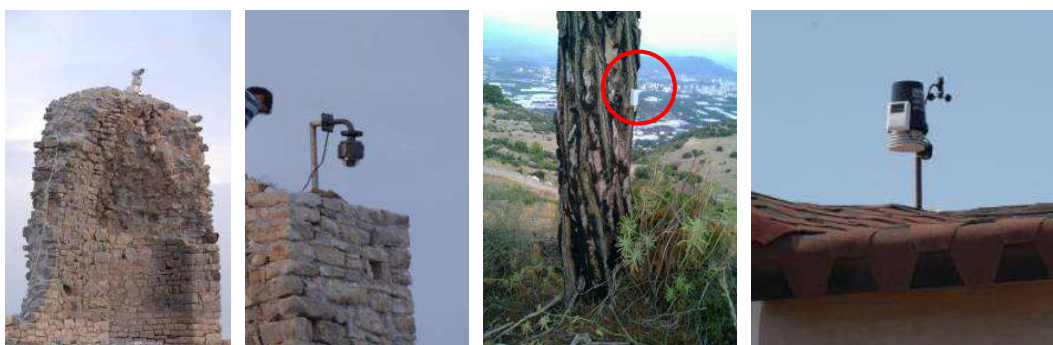
Figure 23: Cameras, WSN node and weather station installed in Rhodiapolis
