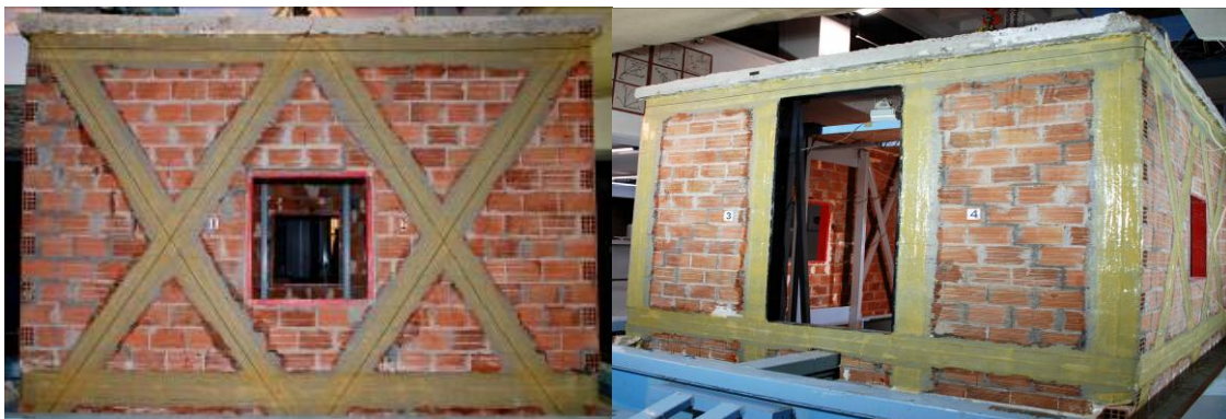
Figure 3.25: The building as reinforced with striped uni-axial textiles. Walls 1 and 2 (left) and 3 and 4 (right)
