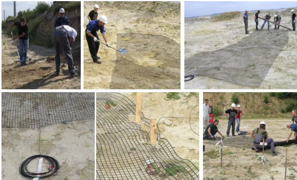
Figure 3.47: Multi-functional geotextile application steps
