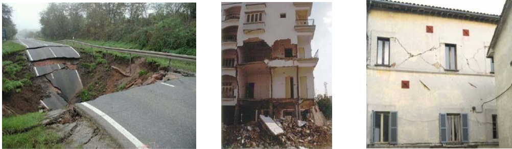
Several views of damage caused by natural hazards
