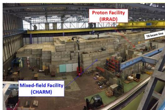
Figure 24: Photo of the irradiation facilities in the CERN East Area. The positions of the facilities behind the shielding and the direction of the proton beam in the T8 beam line are indicated.
