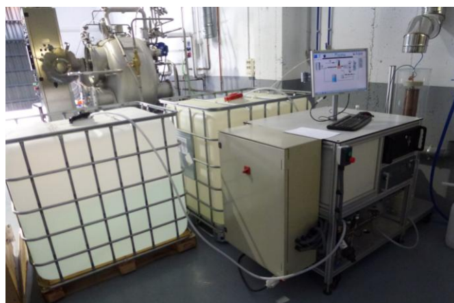
Figure 8: Waterplasma prototype in operation with industrial wastewater from LEBSA
