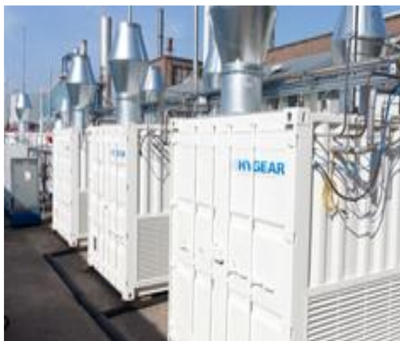
Figure 34. HyGear's (HT&S) on-site hydrogen generation systems: Left: 5 Nm 3 /h system ; Right: 50 and 100 Nm 3 /h system
