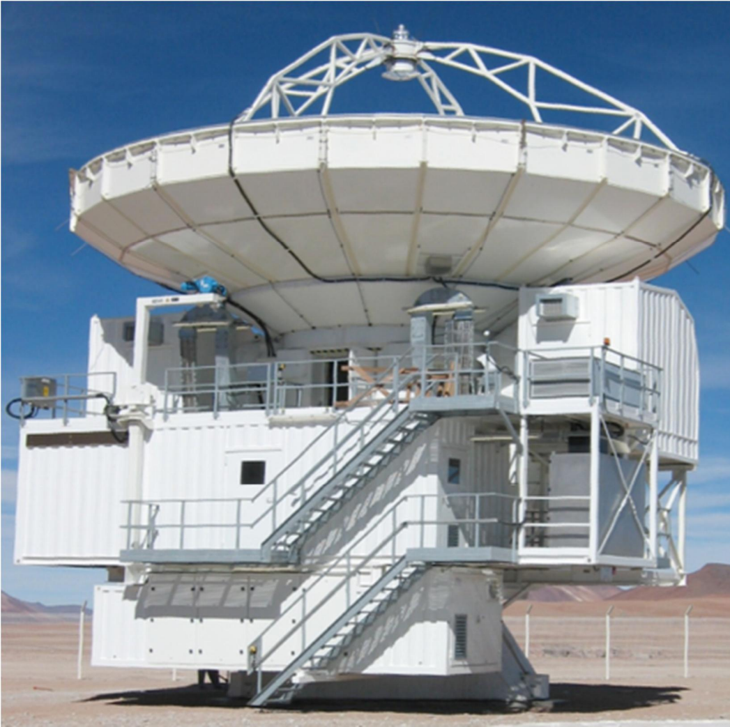
Figure 11: APEX on the Chajnantor plateau at 5100m altitude. The door, seen opened under the dish, is the entrance to the Cassegrain cabin. Only there, a large field of view is available, but not in the cabins around the Nasmyth foci, which are visible on each side.
