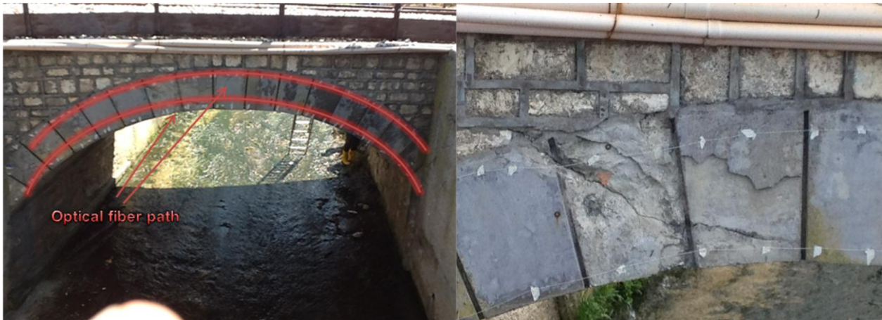
Figure 24 Rail bridge at San Severo-Peschici railway line, near San Menaio Station. It shows cracks at the seaside keystone of the bridge.
