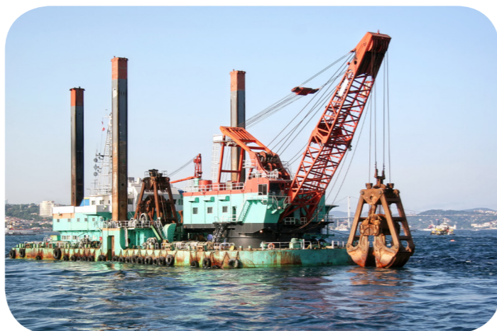
Dredging platform. Dreamstime
