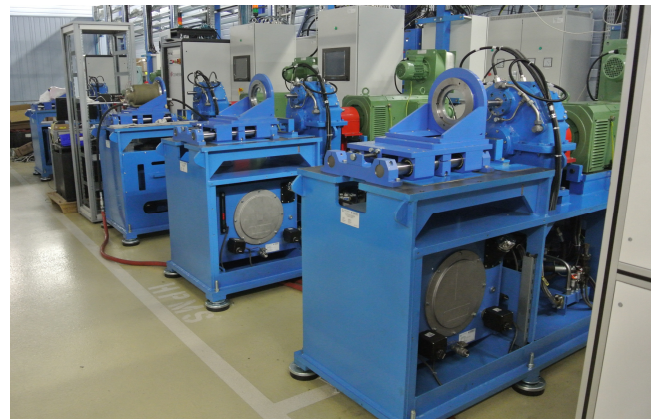
Drives and Control Cabinets
