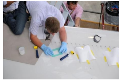
b. Application of paint material
