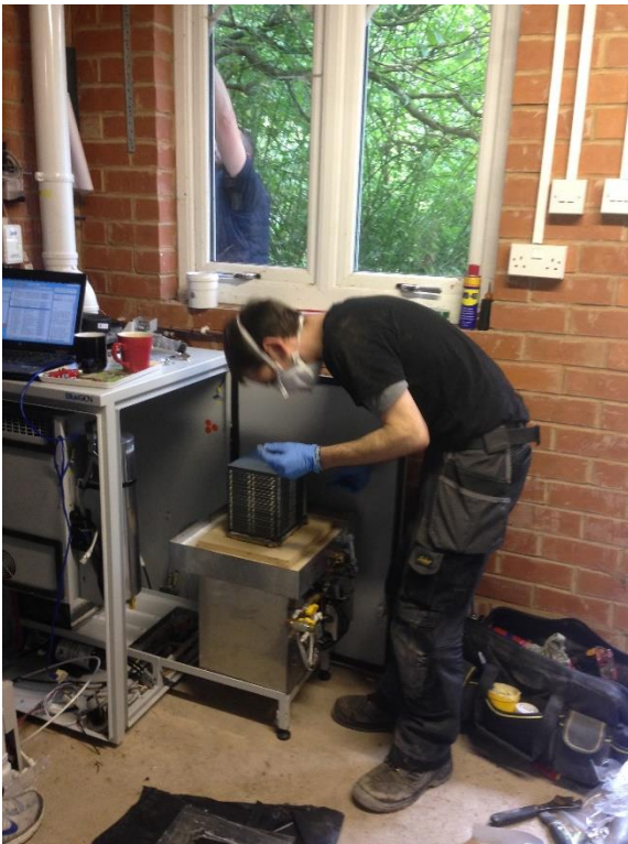
A Stack being installed on site
