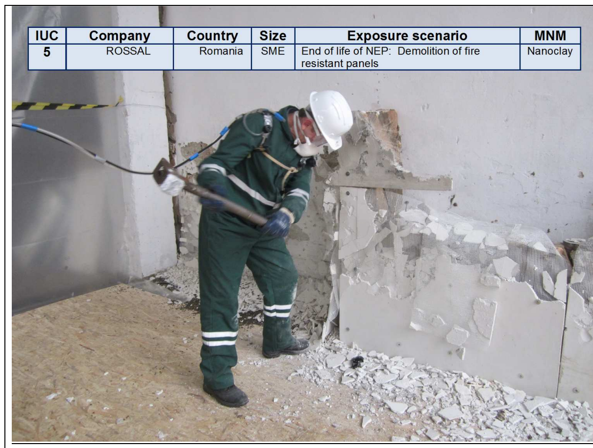
Figure 6.5 IUC5 – Hand demolition with big hammer (10 kg)
