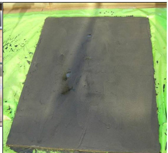
Figure 12: Board covered with rendering plaster
