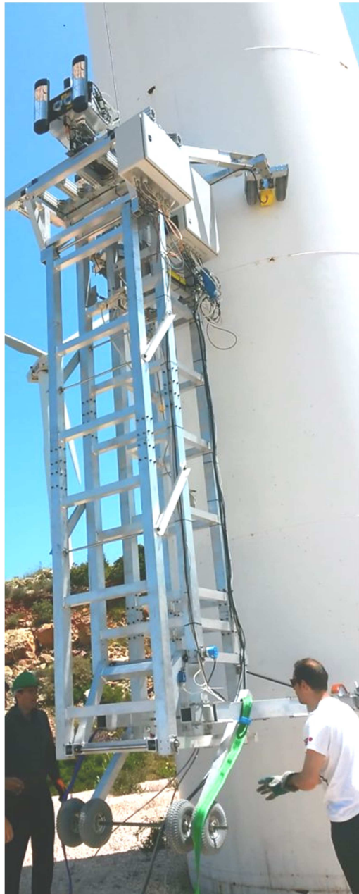
Figure 87 Attachment of the platform on the WTB monopile
