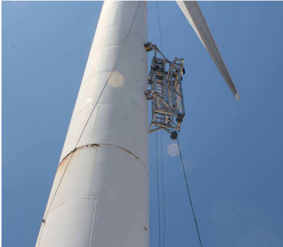
Figure 88 Remote control of the platform to climb up the WTB monopile
