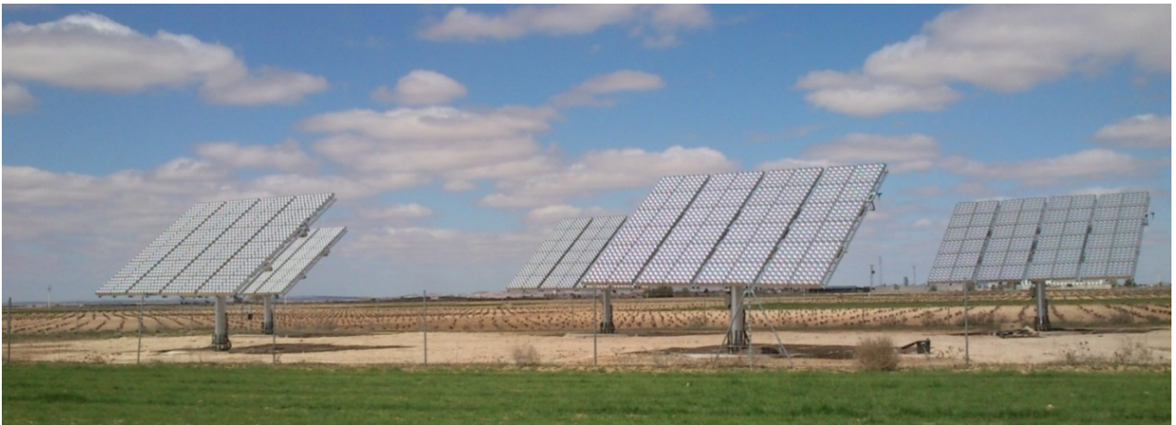
Fig. 15. 50 kWp CPV plant installed at Villa de Don Fadrique. Modules by Daido. Trackers and installation by BSQ Solar.
