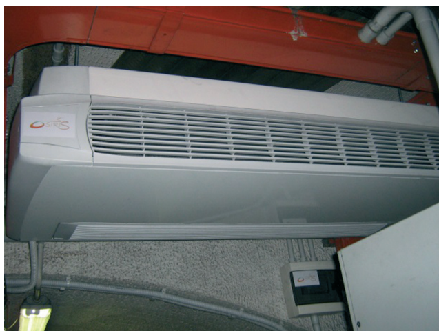
TLC Technical Room Fan Coil
