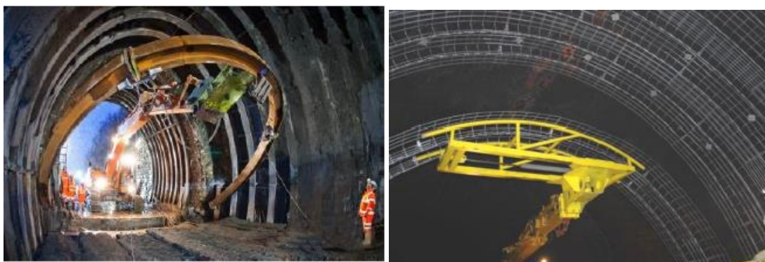
Figure 1-3 Traditional and proprietary tunnel roof support systems
