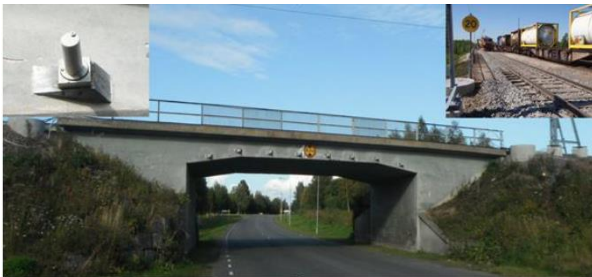
Figure 1-2 The Swedish bridge strengthened with retrospective post tensioning
