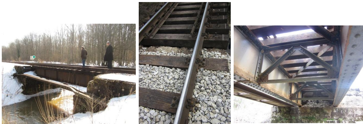
Figure 12: Bunja Bridge in 2012, before rehabilitation
