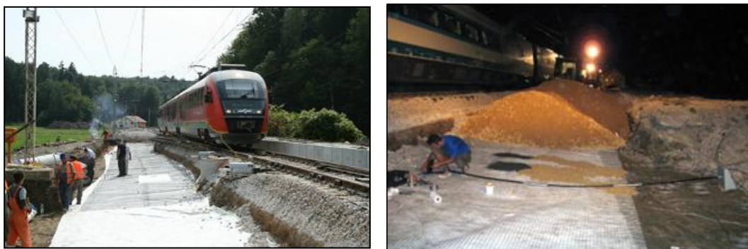
Figure 15; Reconstruction of railway embankment in Dolga Gora site: a) installation of geogrid in combination with a separation and filtration geotextile, b) installation of horizontal extensometer
