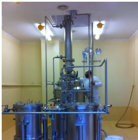
Fig. 7 : Extractor equipment in the Pilot Plant at CTAEX
