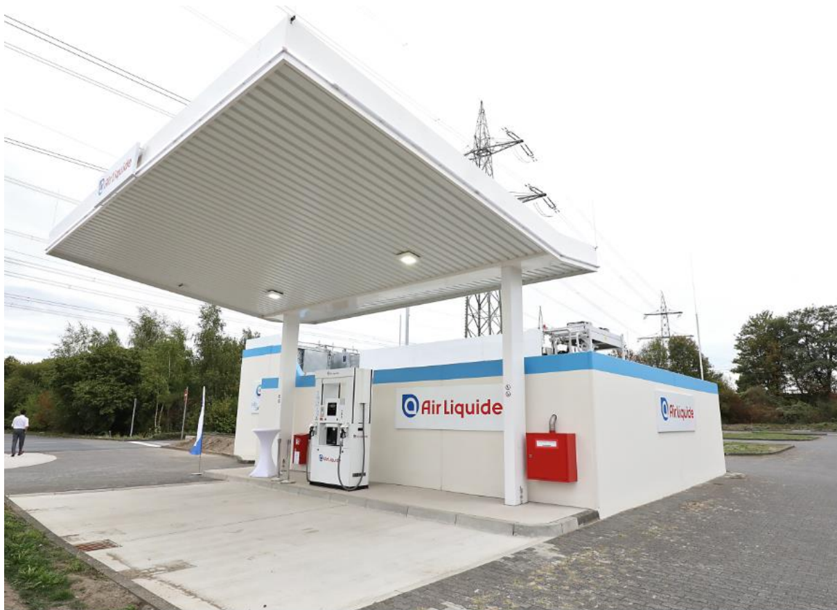
Figure 10 - Finalised Frechen HRS
