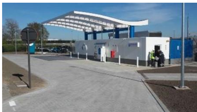
Figure 8 - Air Liquide Zaventem HRS
