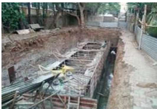
Fig. 7: Construction works for VF constructed wetland
