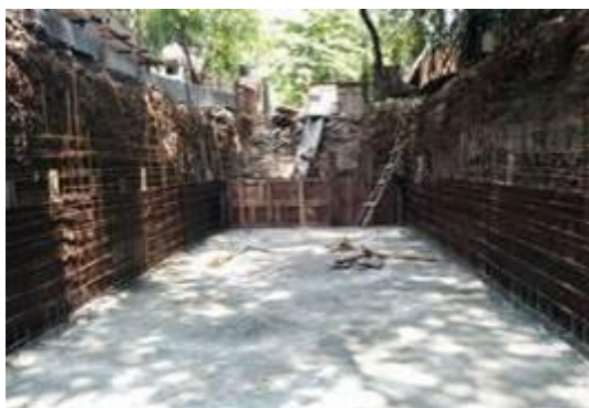
Fig. 5: Construction works for VF constructed wetland and anaerobic treatment at COEP in Pune
