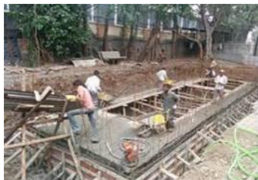
Fig. 8: Construction works for VF constructed wetland and
