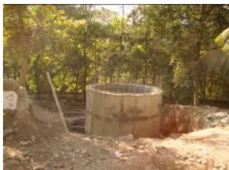
Fig. 55: The intake well under construction at the Indradhanushya Museum site
