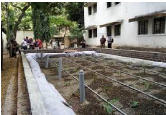
Fig. 25: Greywater system almost completed at COEP in Pune during the EU partners' visit on October 30 th , 2015
