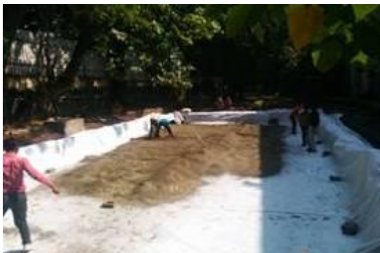
Fig. 23: Water proofing of wetland basins at COEP in Pune
