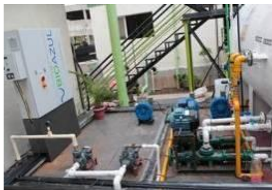
Fig. 4: Wastewater treatment system at Amanora Park Town in Pune – detailed of control panel and connection pipes
