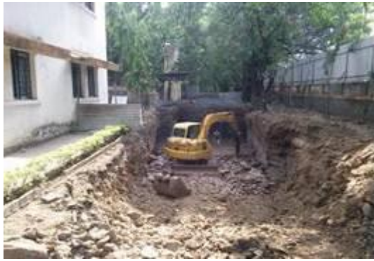
Fig. 9: Excavation works for anaerobic treatment at COEP in Pune
