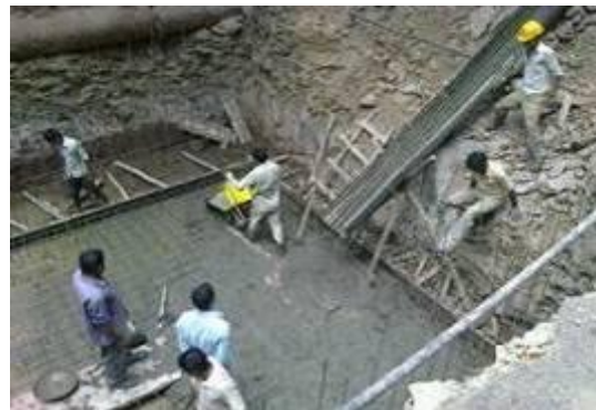
Fig. 12: Preparation of reinforced concrete foundation for anaerobic treatment at COEP in Pune
