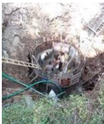
Fig. 56: The intake well under construction at the Indradhanushya Museum site
