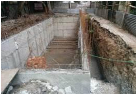
Fig. 13: Construction works for anaerobic treatment (left) and constructed wetland (right) at COEP in Pune
