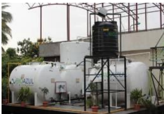
Fig. 3: Wastewater treatment system at Amanora Park Town in Pune – installed MBR and SBR systems
