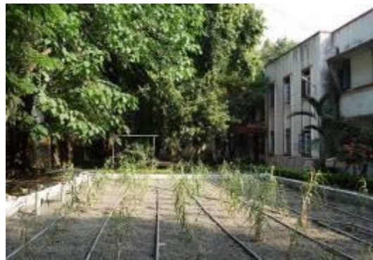
Fig. 26: One of the 3 tertiary treatment VF CW systems at COEP in Pune in December 2015
