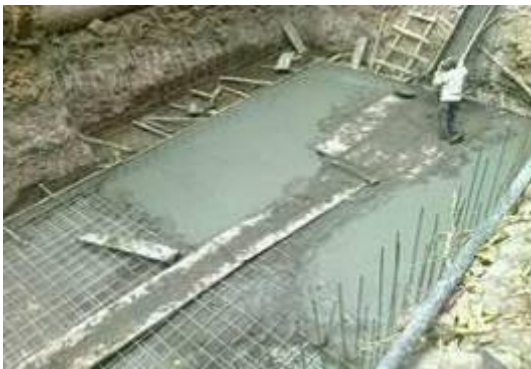
Fig. 11: Preparation of reinforced concrete foundation for anaerobic treatment at COEP in Pune
