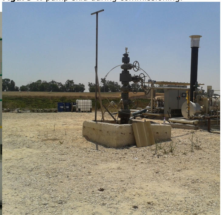
Figure 6: Connection to the injection well.
