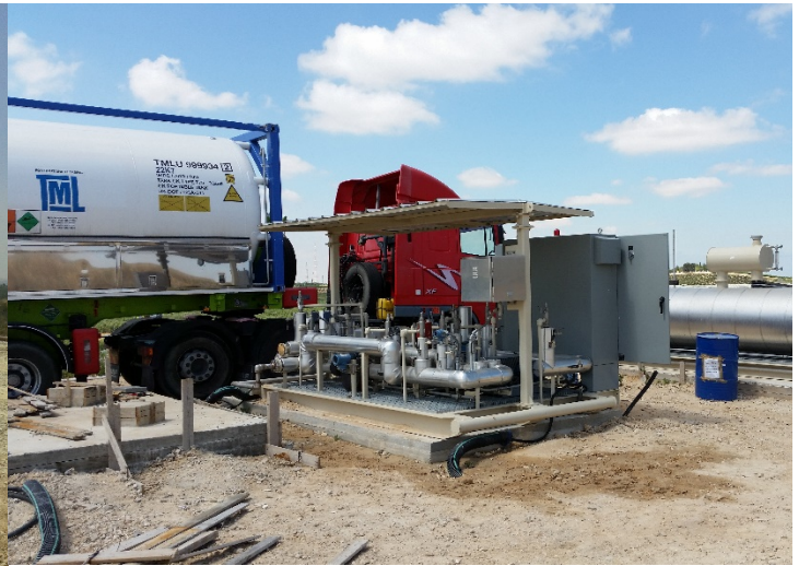
Figure 4: pump skid during commissioning.
