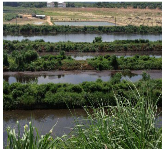
Figure 2. POME purification ponds in Thailand, Particulate matter is allowed to settle before the water is pumped over farmland.
