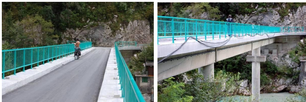
Figure 38 The bridge after the rehabilitation.
