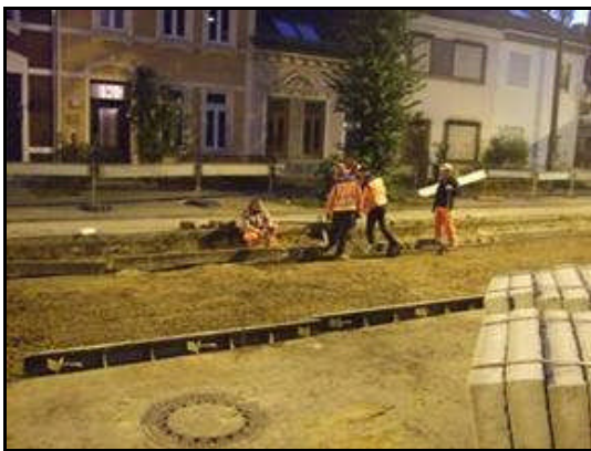
Installation of shuttering and adjustment
