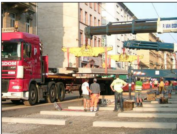
Assembly of track slabs
