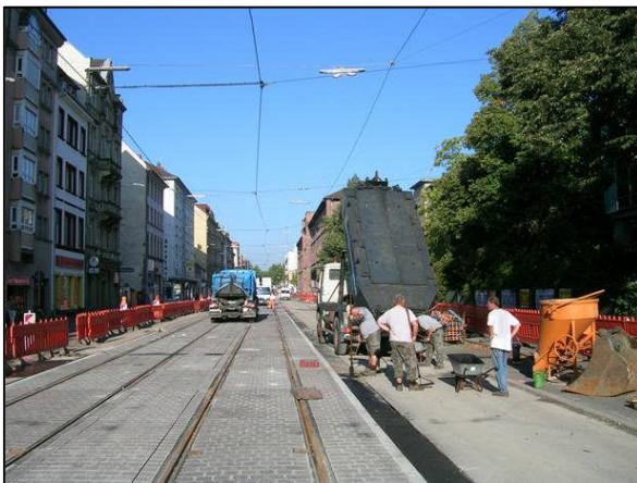
Asphalting the road edges
