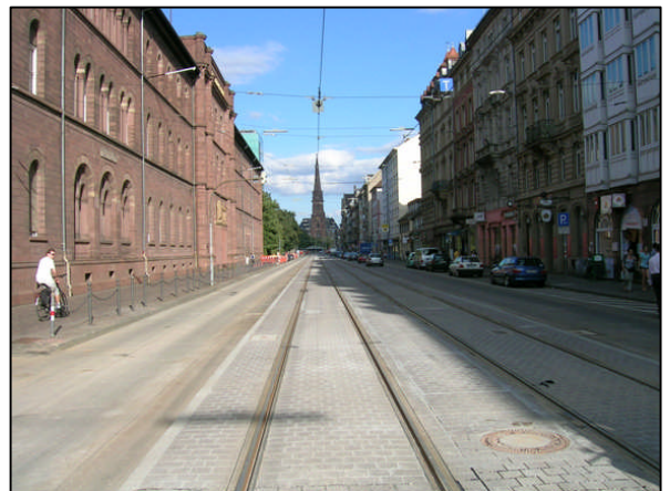
Construction site done
