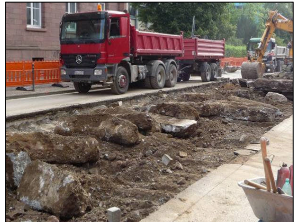
Removal of base plates
