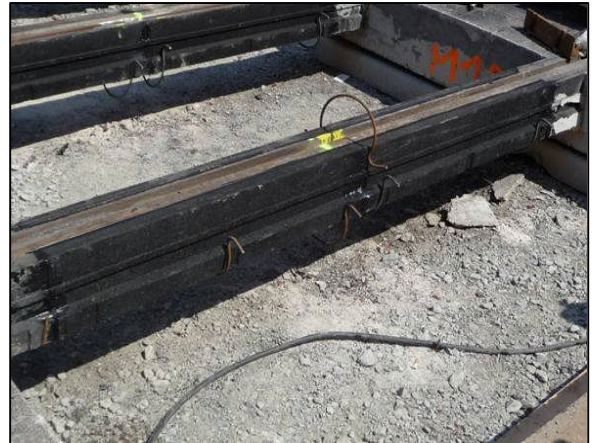
Jackets at the welding zones
