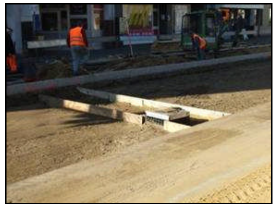
Disassembling of the base layer and preparation and compaction of formation level
