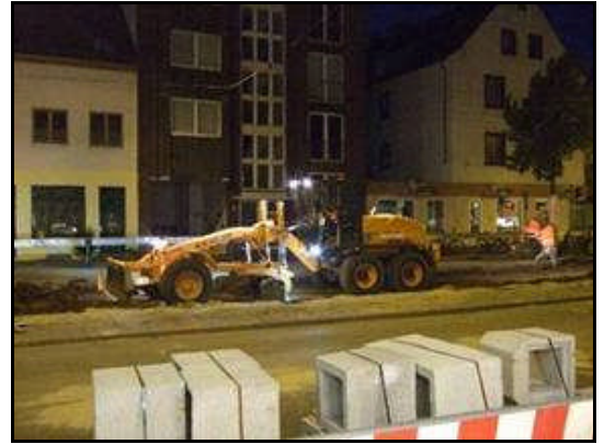
Disassembling of the base layer and preparation and compaction of formation level
