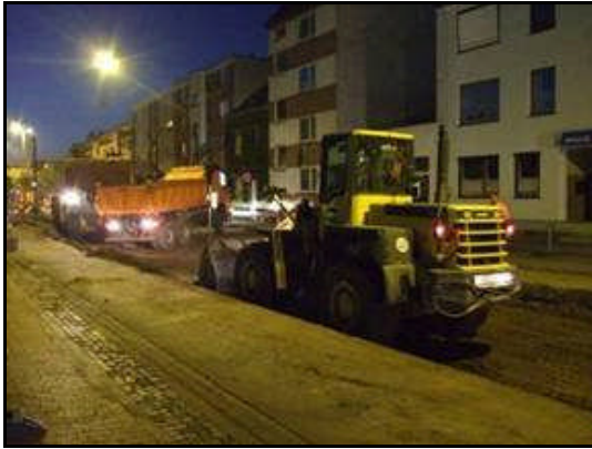
Disassembling of the base layer and preparation and compaction of formation level
