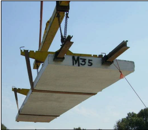
Unloading track slab elements at the harbour of Karlsruhe
