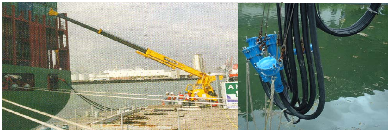
Examples of state of the art cold ironing connections
