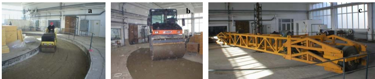
Figure 3 Construction of the trial LLRP (a and b) at ALT LIRA facility (c)
