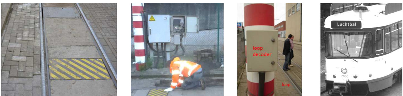
Figure 5- Wayside axle bearing monitoring system for Light Rail Vehicle
