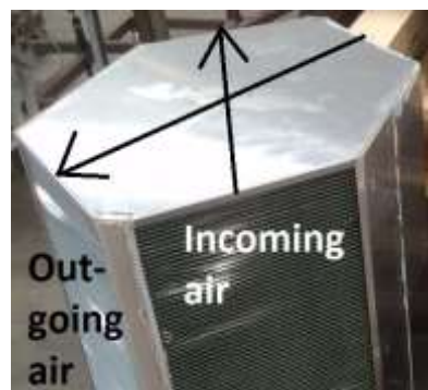
Figure 5: Aluminium counter-flow plate heat exchanger for heat recovery ventilation.
