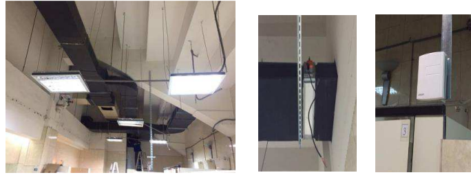
Figure 29. Air ducts installation, damper and sensor
