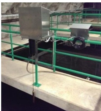
Figure 12 Left: Installation of the CBX sludge level meter at Bromma WWTP. Right: Example of a sludge concentration profile in the secondary sedimentation tank. The red line is an example of a critical profile.
