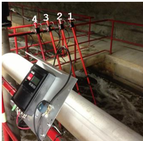
Figure 8 Installation of the four DO sensors at the Bromma WWTP
