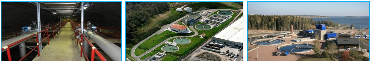
Figure 2 The Bromma WWTP (left), the Mekolalde WWTP (centre) and the Mussalao WWTP (right), plants where DIAMOND Systems have been tested and validated
