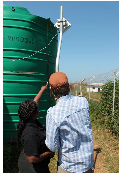
Researchers from Fraunhofer FOKUS assisting in the setup of a WiMax CPE to provide Internet access to Lurwaizo SS school in Dwesa.
