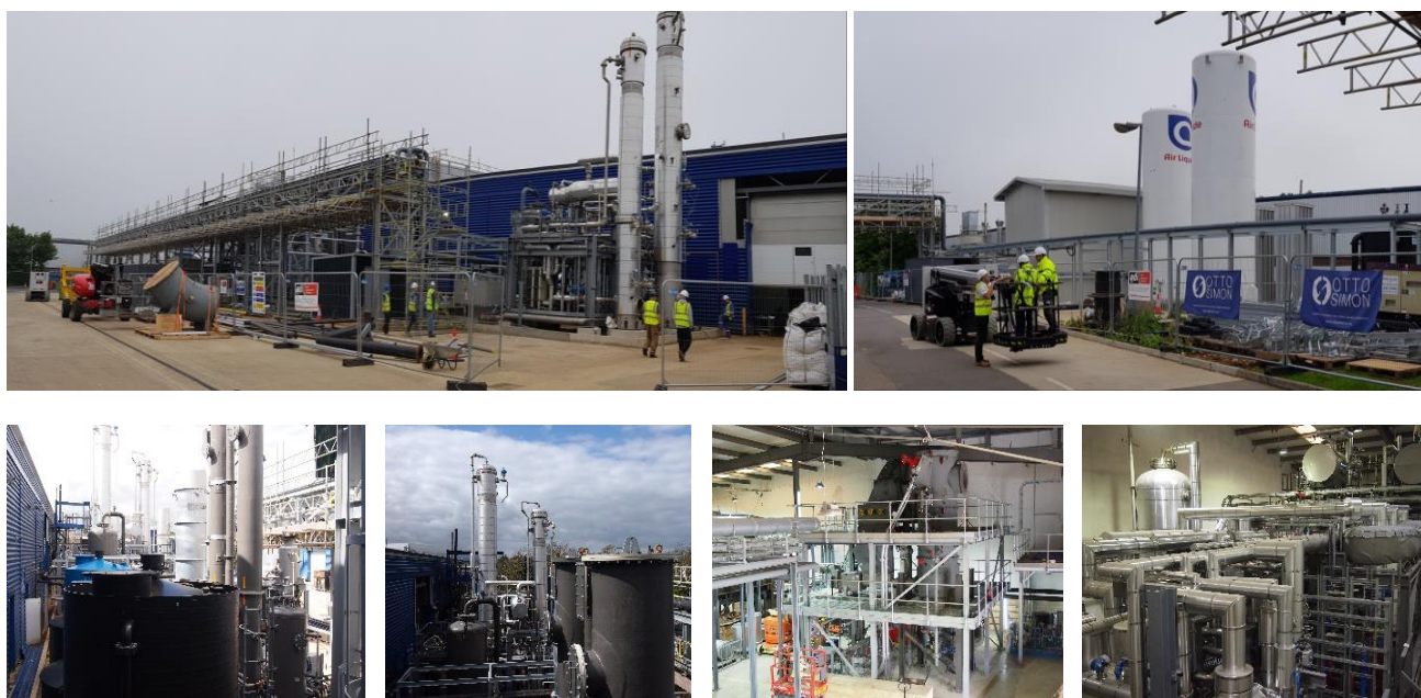
10,000 tonne per annum scaled up plant under construction, based on the BESTF support facility
