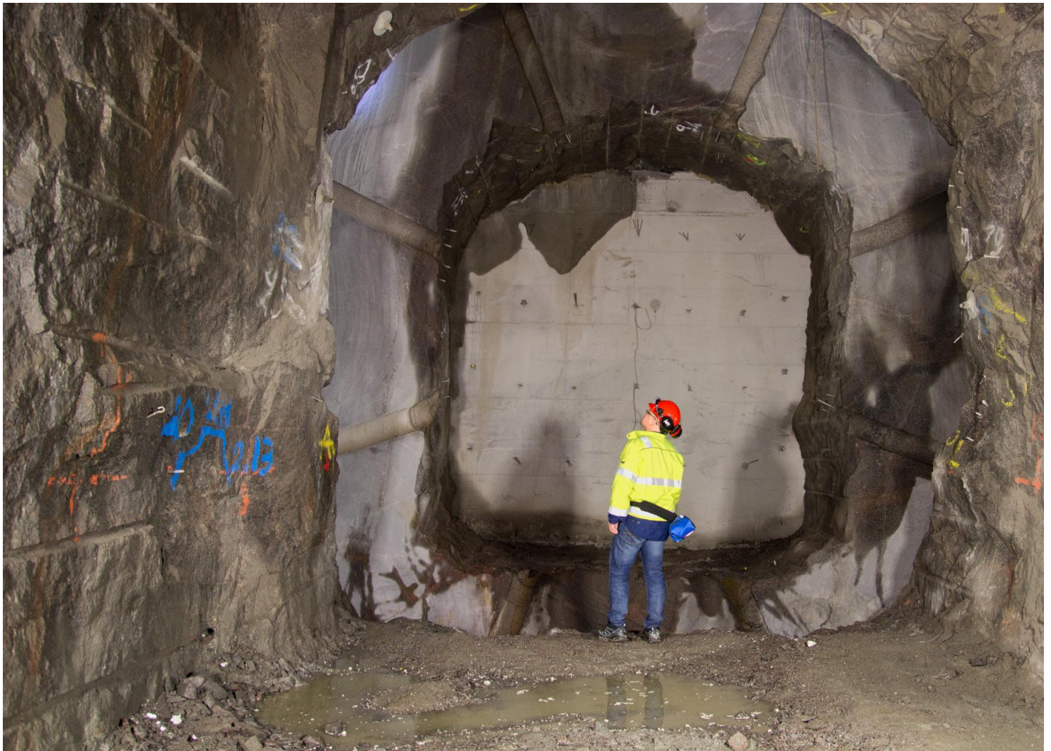
The DOMPLU (one of the DOPAS full scale experiments) plug location in crystalline host rock based on laser scanning in 3D model and the plug location in reality after wire sawing in Äspö Hard Rock Laboratory in Sweden. Photo: SKB
