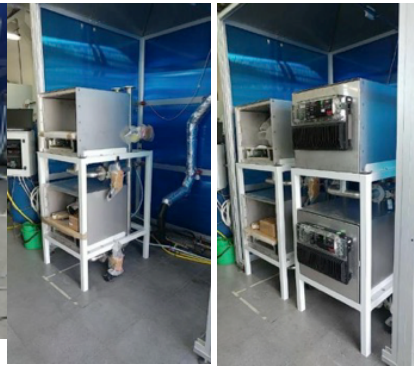
SNC batteries installation and test
