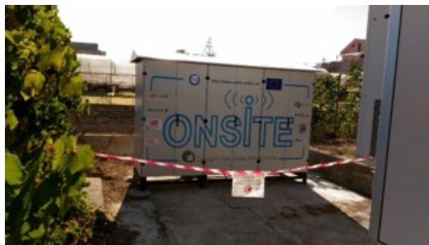
Figure 27: The developed system at the field trial site
