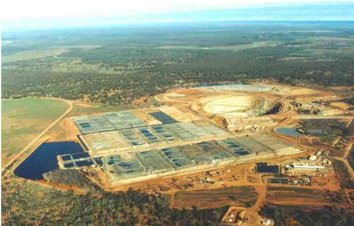
Figure 14: Copper heap bioleaching operation showing mining pit and heap bioleaching pads.
