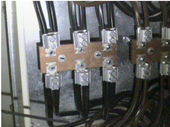
Fig.: Digital and IR pictures of a cable connection cabinet. If there was something wrong with one of the connections, the IR-Image would show a temperature difference within the different phases.
