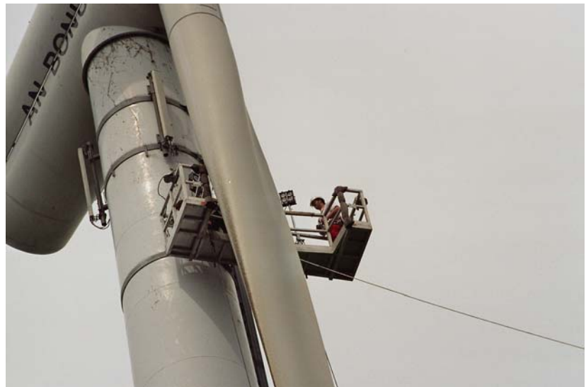
Fig.: with the platform it is very easy to move up and down with the PREWIND system.
