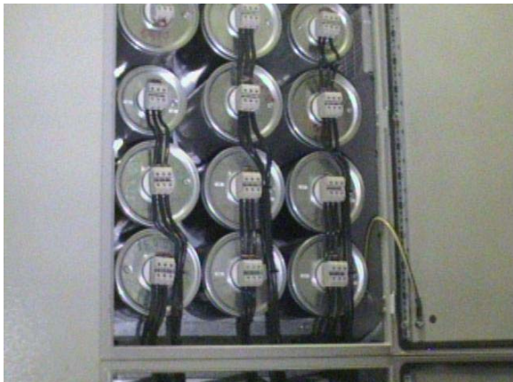
Fig.: Digital and IR pictures of the electrical cabinet A4 (the compensation cabinet). The thermogramme shows clearly which circuits are working and which not.
