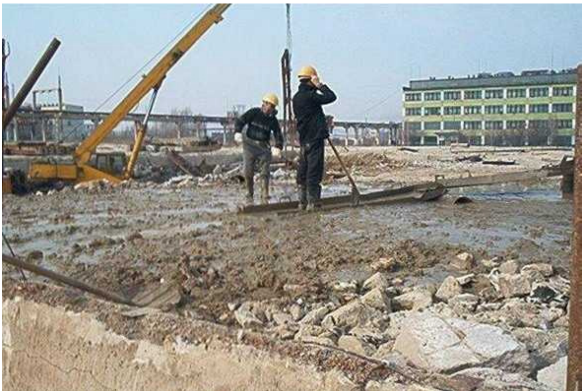
Fig.23. Filling in the first compartment of the landfill with ground-concrete mixture
