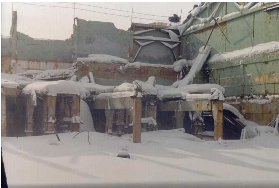
Fig.16. Building 31 – electrolysis shop (northern side) after dismantling the roof, winter 1998/99.
