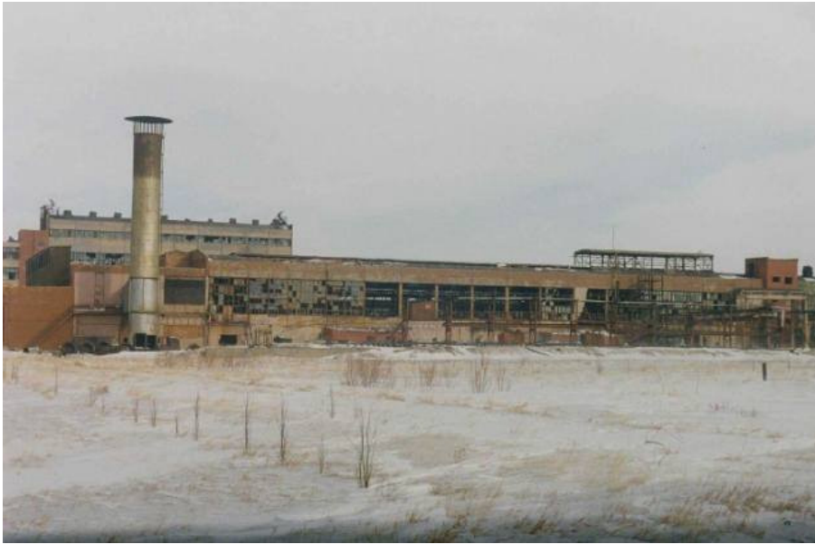
Fig.14. Building 31 – electrolysis shop (southern side) before demolishing the building, winter 1998/99.
