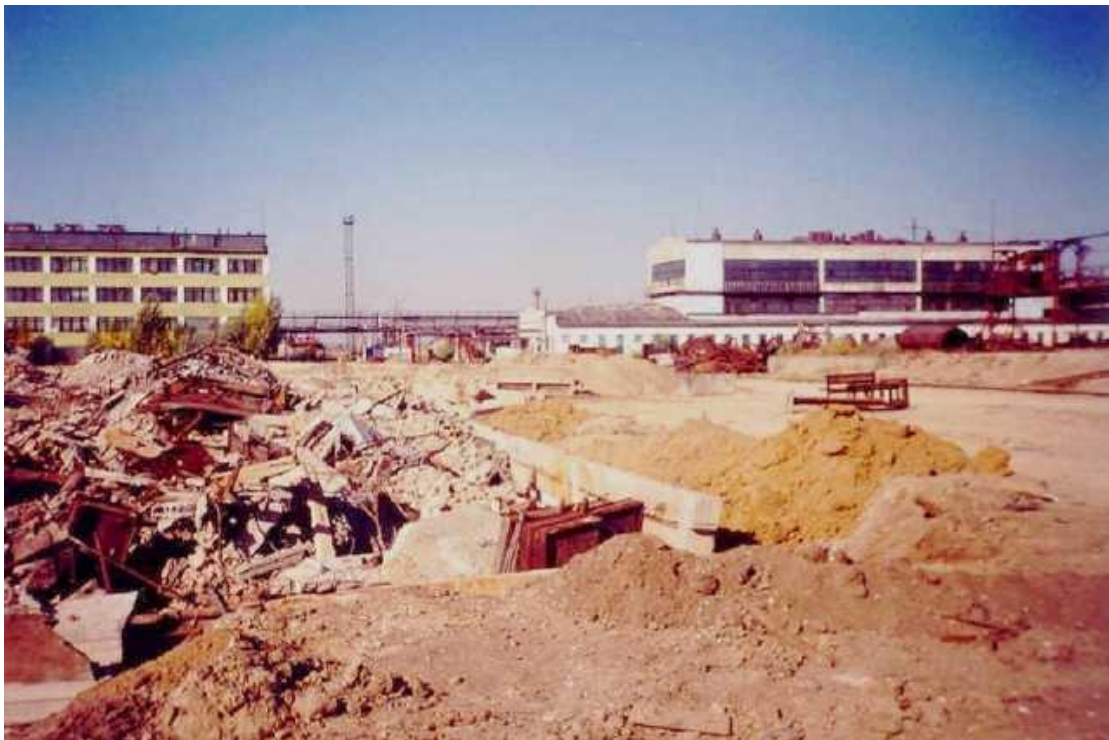
Fig.21. Piling mercury contaminated building structures into the first compartment of land-fill
