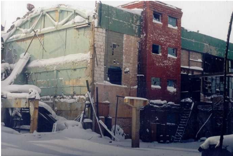
Fig.15. Building 31 – electrolysis shop (northern side) after dismantling the roof, winter 1998/99.
