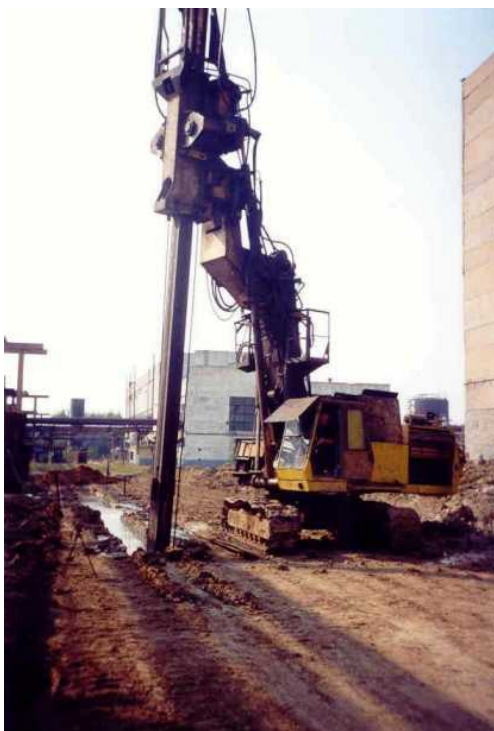
Fig.17. Construction of anti-filtration screen, so called cut-off wall around the building 31
