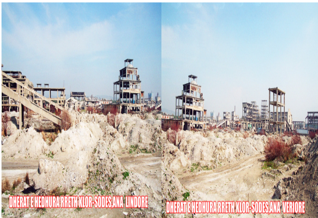
(a) East part of the Plant
