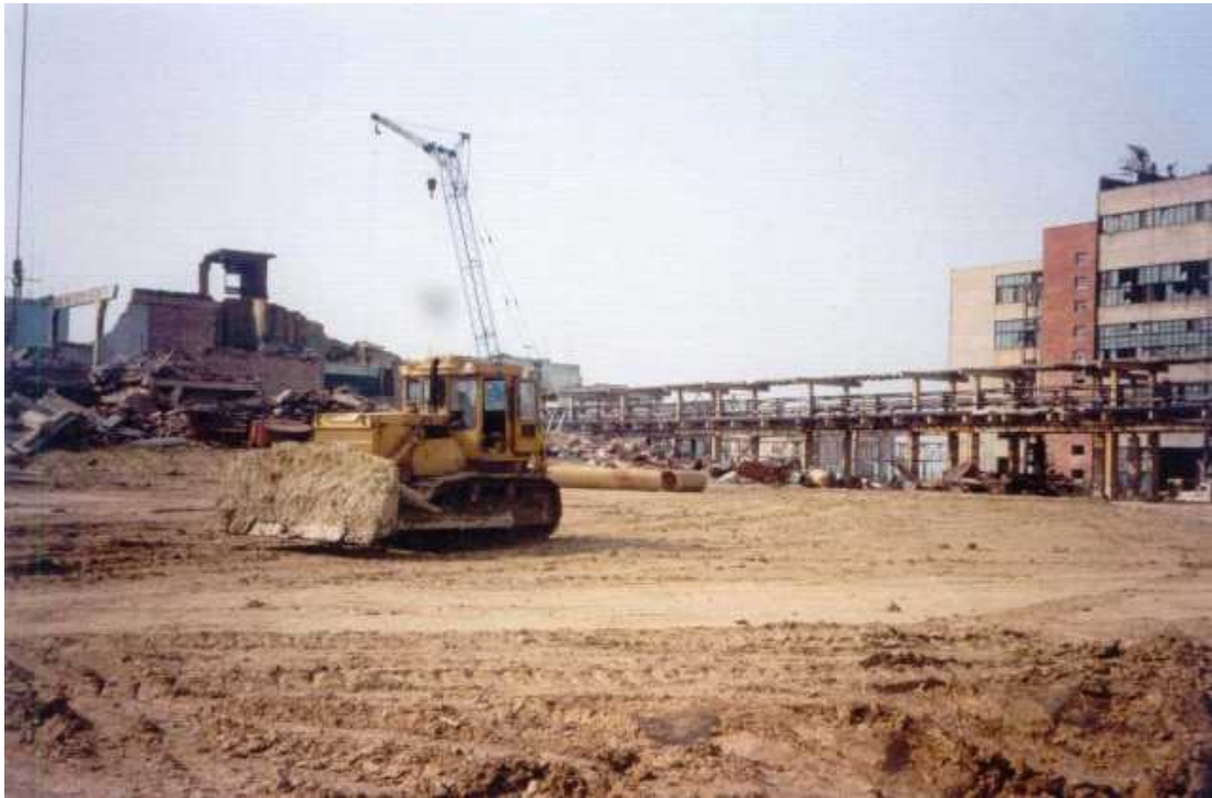
Fig.20. Creation of clay covering above the concrete foundation of the building 31
