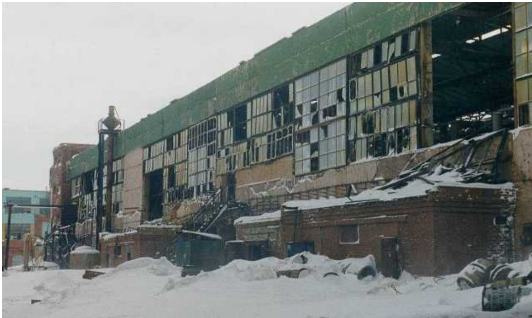
Fig.13. Building 31 – electrolysis shop (northern side) before demolishing the building, winter 1998/99.
