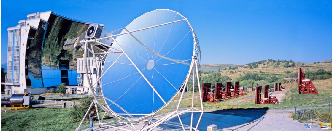
Figure 3: The 50 kW solar dish (SDISH 50kW)
