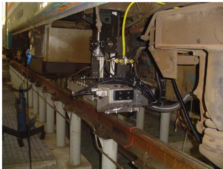
Detail of equipment under the rail vehicle
