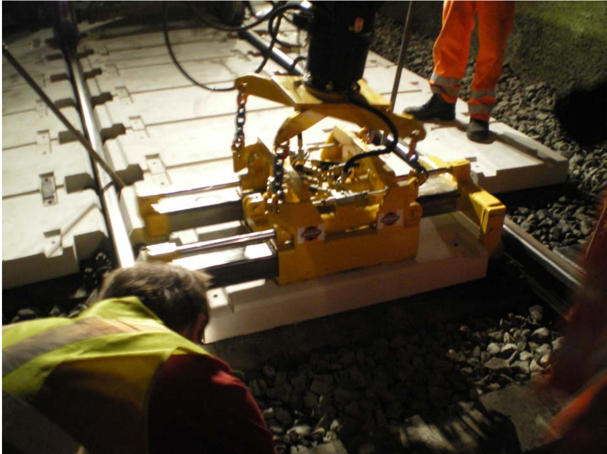
Fig. 5. Process of the installation of the CORPTUS panels.
