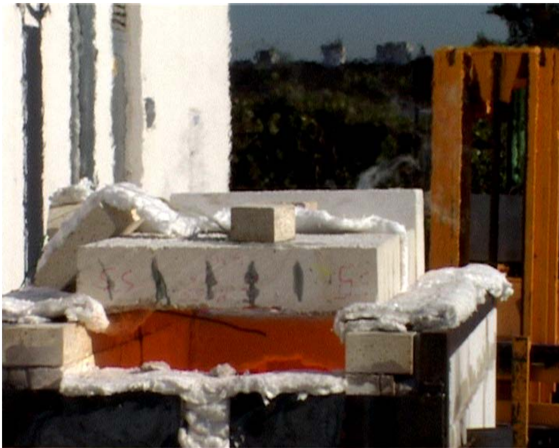
Fig. 3: Preparation of large scale concrete models for fire tests
