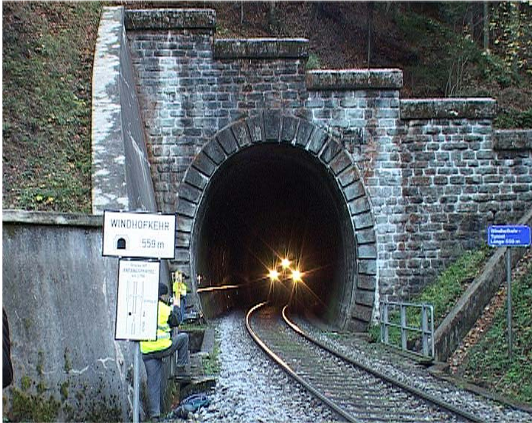
Fig. 2: The test tunnel Windhofkehr in Austria
