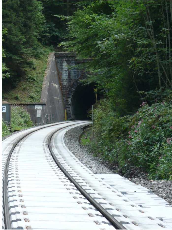
Fig.6 Corptus panels installed in the access into the tunnel.
