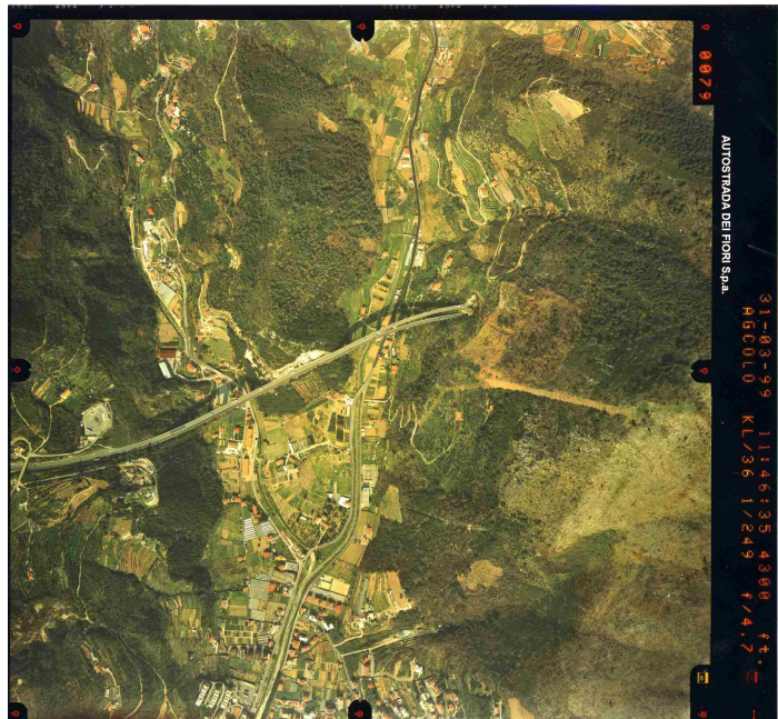
Figure 47 Aerial view – Viaduct of Maremola
