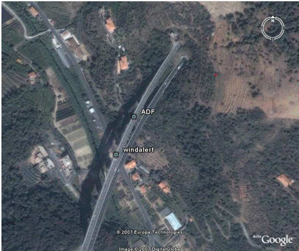
Figure 47a: Location of the WindAlert system and the ADF station on the Maremola viaductAerial view
