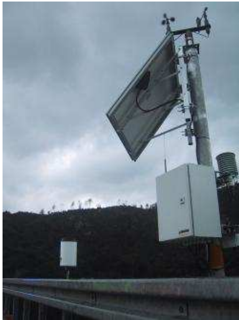
Figure 46 WindAlert prototype on the viaduct of Maremola
